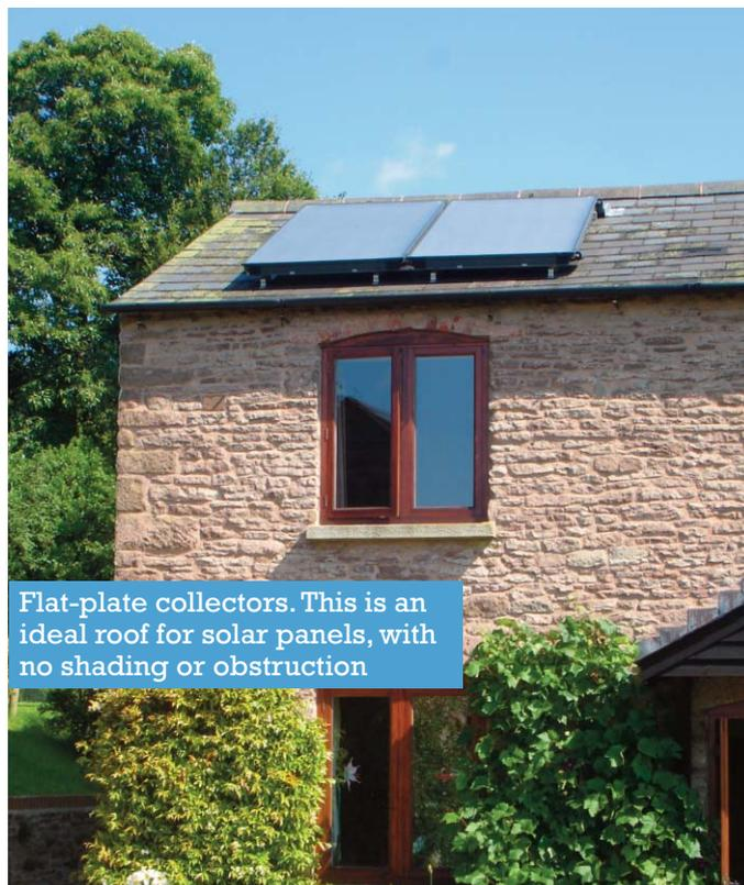
Flat-plate collectors. This is an ideal roof for solar panels, with no shading or obstruction
